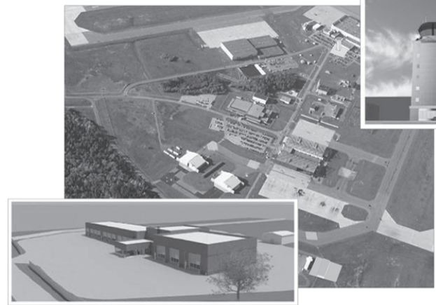
Refueling Tender Garage
