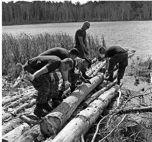
The RAS team made use of the trees felled during chain saw training to piece together a rough dock for Camp Aldershot training use.
